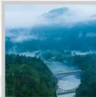
"TADAMI FIRST BRIDGE"
